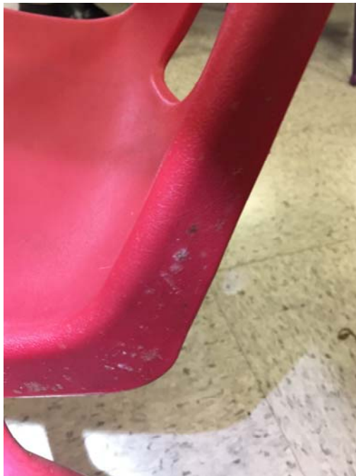
Photo 32 – Kindergarten Room 3 Mold growth was observed on the plastic chairs.
