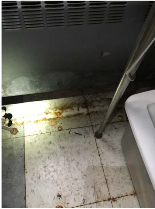
Photo 27 – Kindergarten Room 2 Closet
