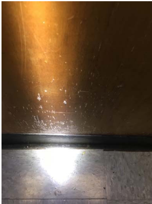
Photo 20 – Kindergarten Room 2 Mold growth was observed on the built-in wooden cabinetry and coat cubby.
