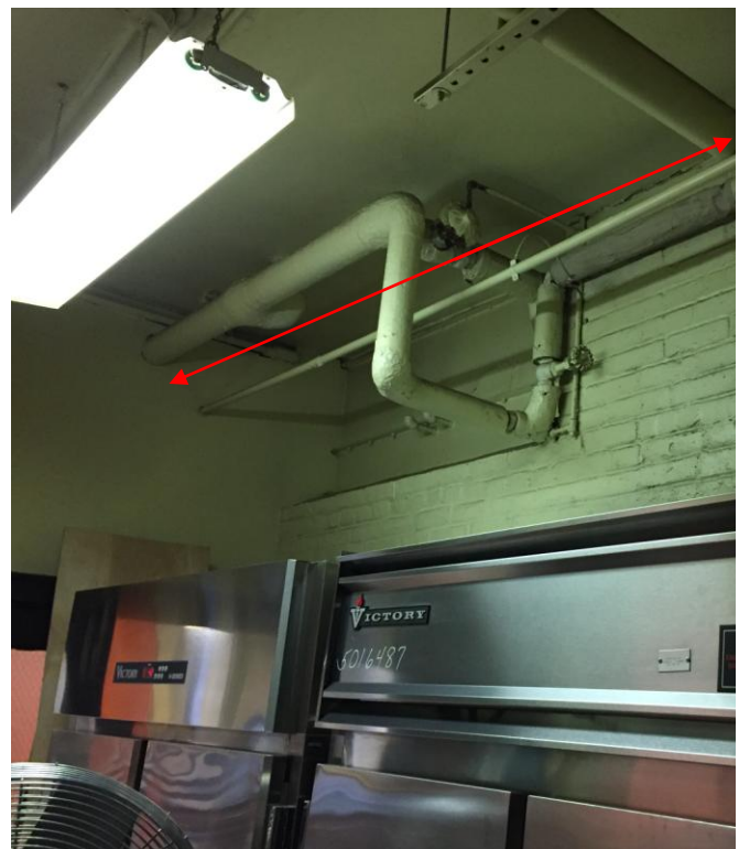
Kitchen Area – Adjacent Hallway above 2 Small Freezers Remove 13 LF of damaged ACPI and 8 ACPFs (laterals above freezers) - Minor Project
