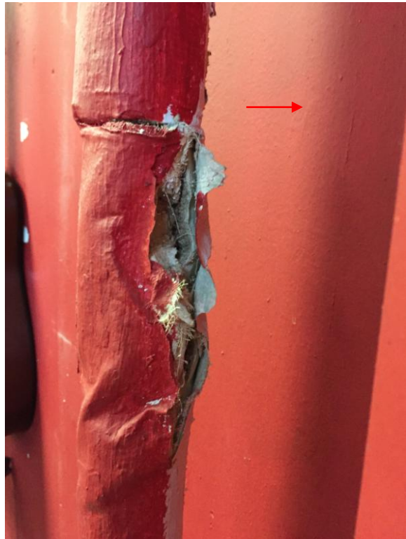
133 – Music Classroom 133 Remove 14 LF of damaged ACPI (riser beside left hand rear corner) - Minor Project Outer lagging is ripped and torn
