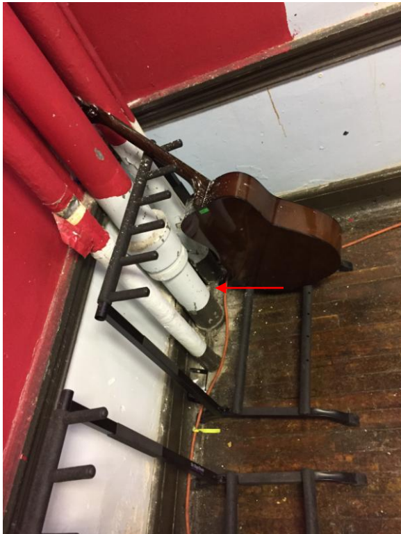
133 – Music Classroom 133 Remove 14 LF of damaged ACPI (riser beside left hand rear corner) - Minor Project Outer lagging is ripped and torn
