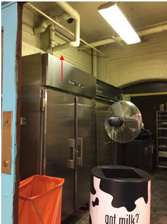
Kitchen Area – Adjacent Hallway above 2 Small Freezers Remove 13 LF of damaged ACPI and 8 ACPFs (laterals above freezers) - Minor Project
